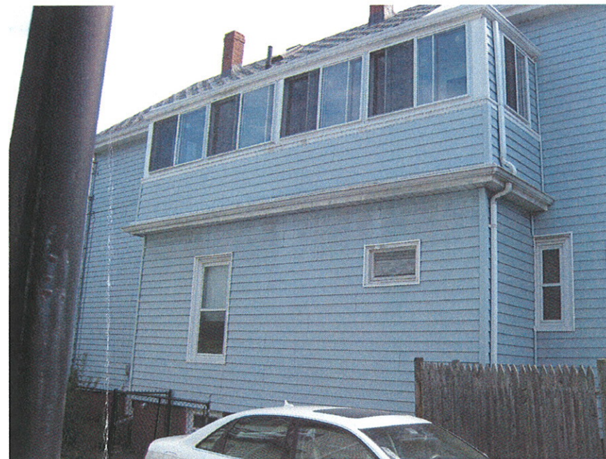
VIEW OF EXISTING EAST ELEVATION / LOOKING SOUTHWEST
