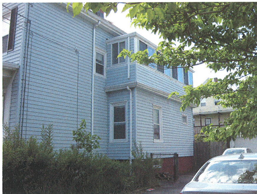
VIEW OF EXISTING EAST ELEVATION / LOOKING NORTHWEST
