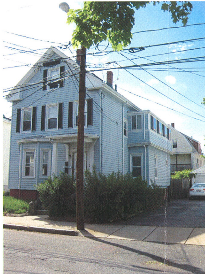
VIEW FROM IRVING ST. / LOOKING NORTHWEST
